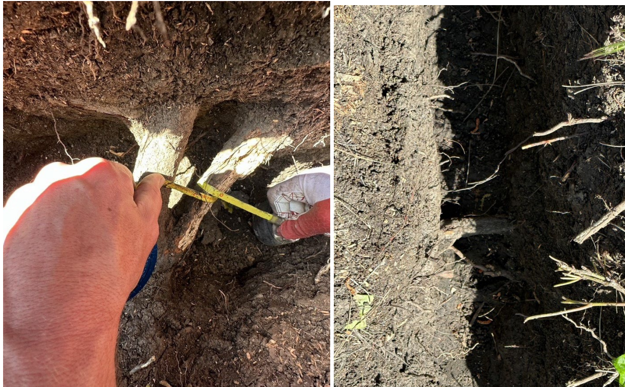
Showing the two 2" diameter roots encountered at the pool house foundation
