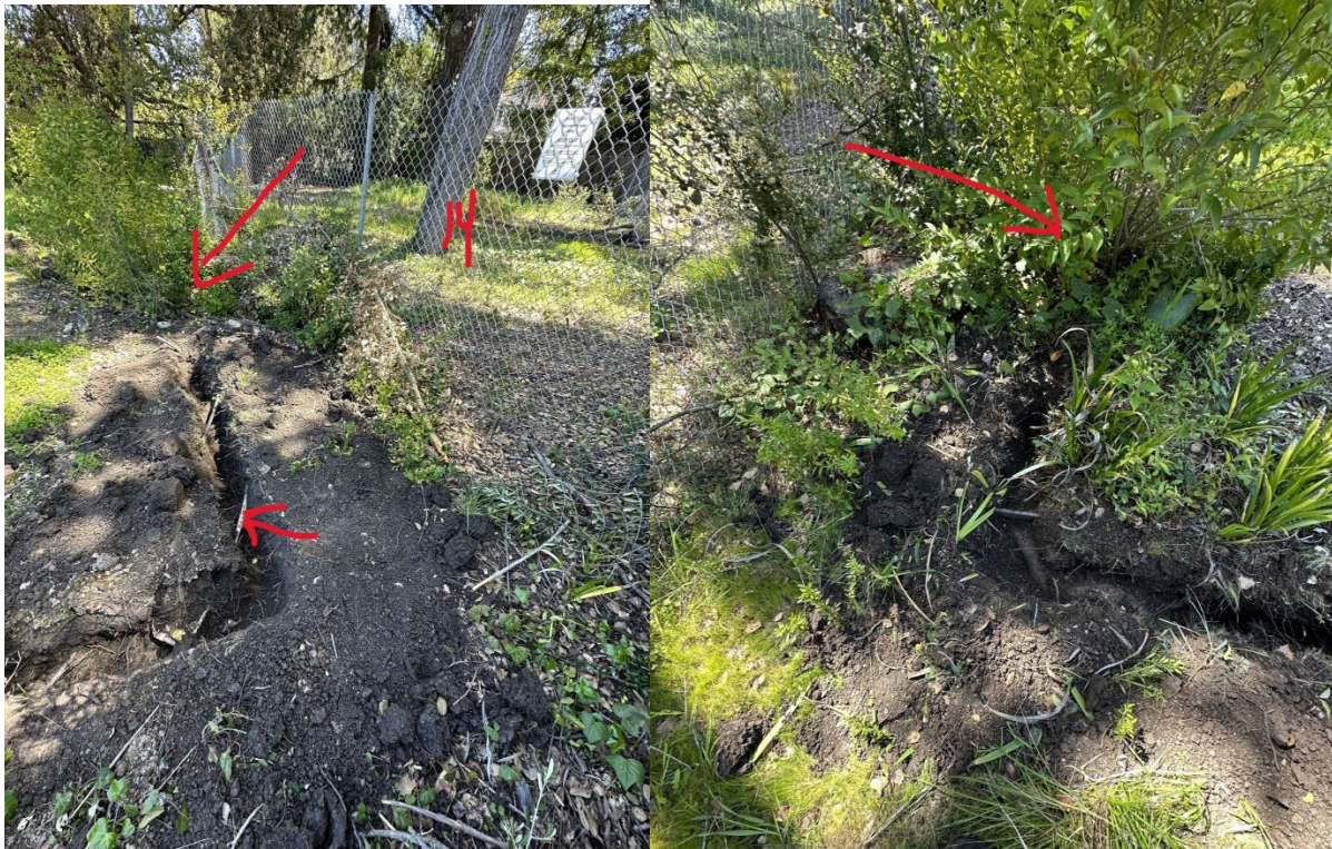
Showing exploratory trench at home foundation near oak tree #14, red arrows showing large stump and irrigation lines encountered
