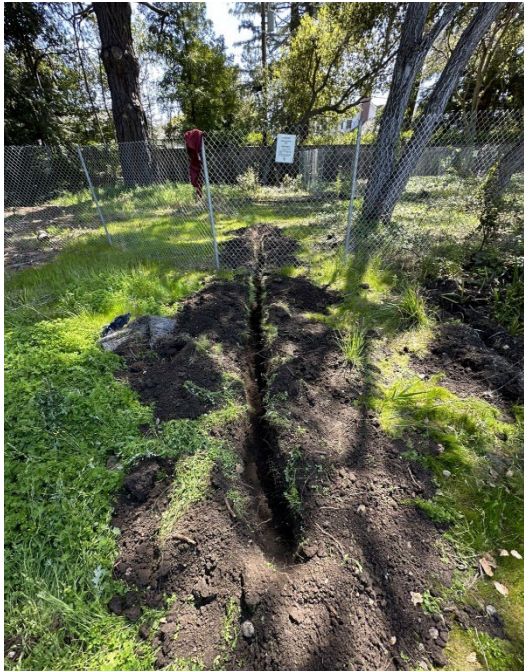
Showing exploratory trench near oak tree #14 for the decomposed granite area
