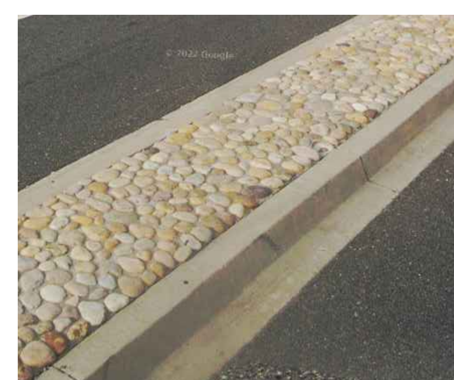
RIVER ROCK PAVING DETAIL "E" NTS
