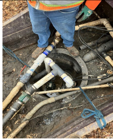
Playground bathroom pump repair
